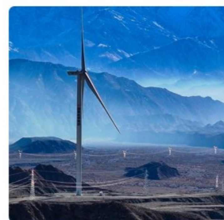
Wind Power Generation
